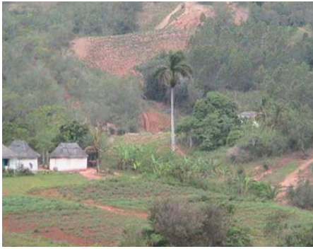
Figure 2. Effects of erosion in UME “Ceja del Río”. Section I -I. (Source: self-made)
